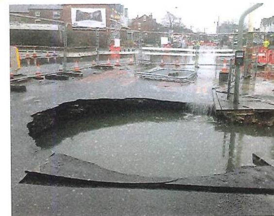
Figure 13.13 Collapsed sewer in Southport.
